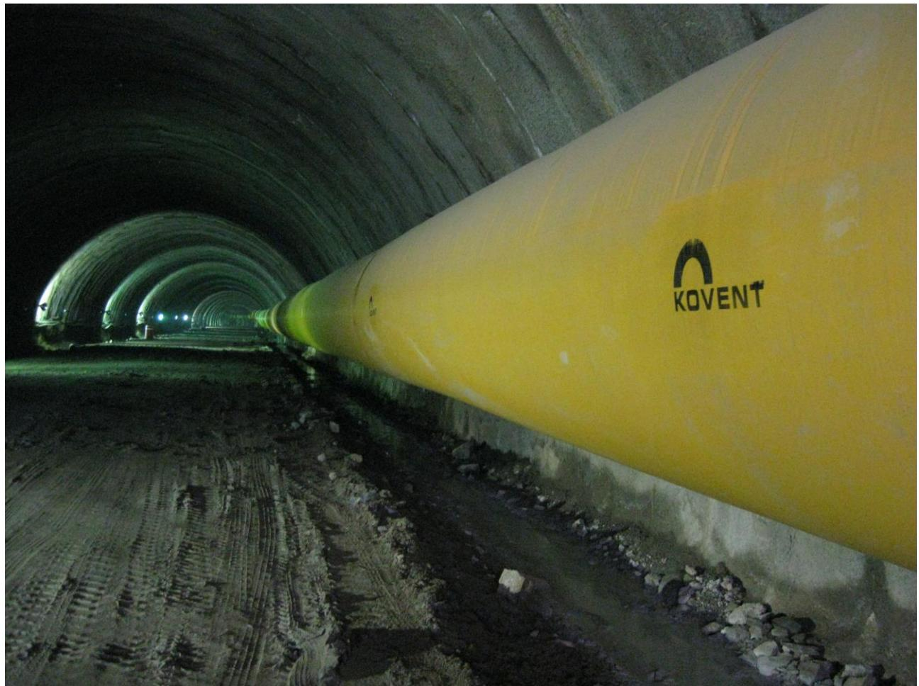
**KITEX FLEXIBLE DUCTING** is manufactured from PVC Coated Polyester Fabric and is distinguished by the relatively low weight with kept high strength values which results in a very pliable and easy to handle duct.
